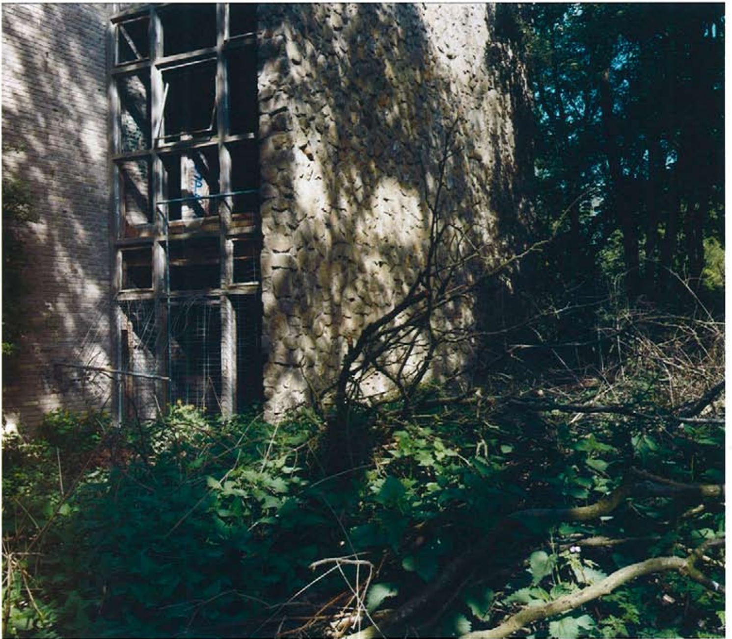
8. The rubblestone wall at the back of the stage building
