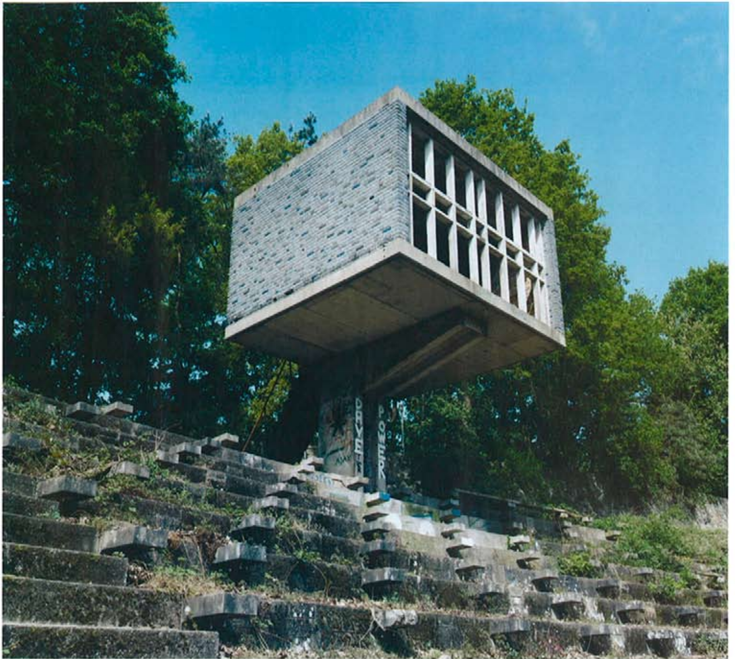
10. The cantilevered 'box' from which performances in the theatre were directed
